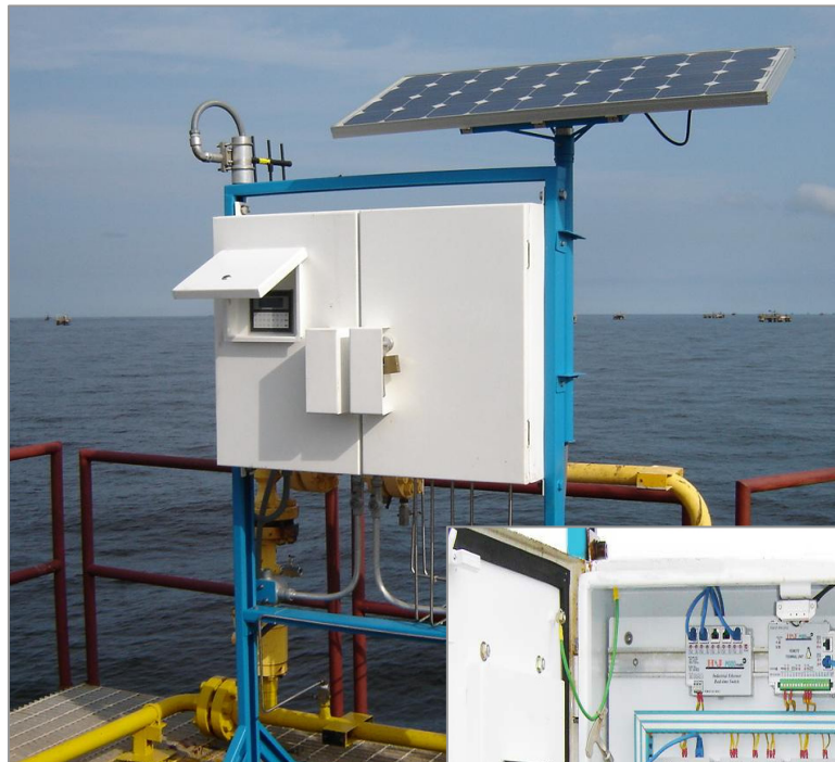
POZomatic Control Cabinet Exterior and Interior Views
